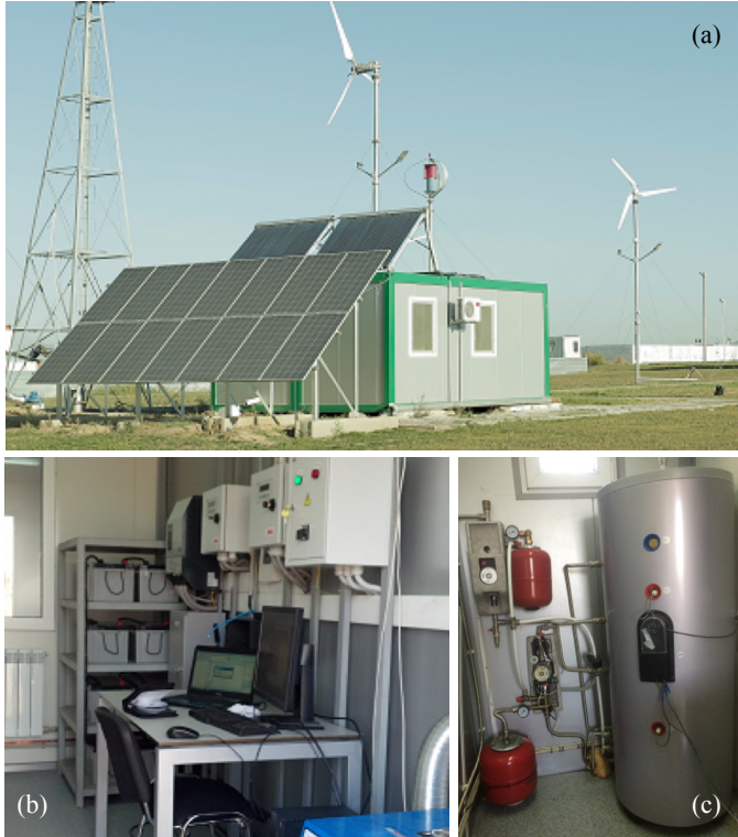
Figure 1: (a) exterior of the smart house, including PV panels and solar collectors; (b) interior, including control computer, battery pack and charge controller; (c) interior, including thermal storage tank and pumps
